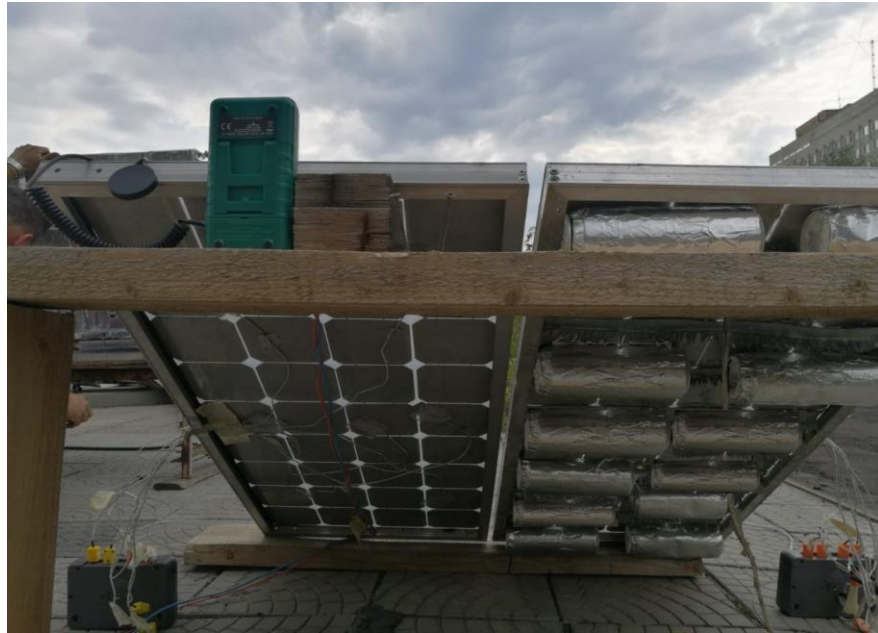
Fig. 5.13 Rear side of the PV panels: referenced (left) cooled (right)
