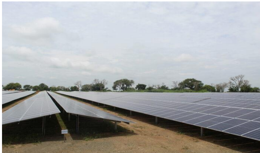
Fig. 1.3 Lawra solar power plant [4]
